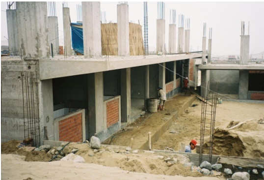
San Jose under construction in 2006
