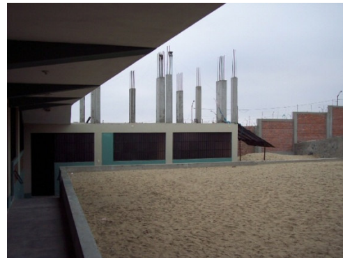
San Jose in 2007, ready for 2 nd floor
